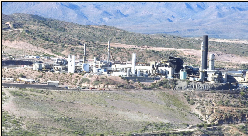
FIGURE 13 ACID PLANT This is in Globe-Miami -- I believe that this is the acid plant. There, sulfur trioxide gas captured from the smelter, is processed into sulfuric acid, used in heap leaching of oxide ores.
