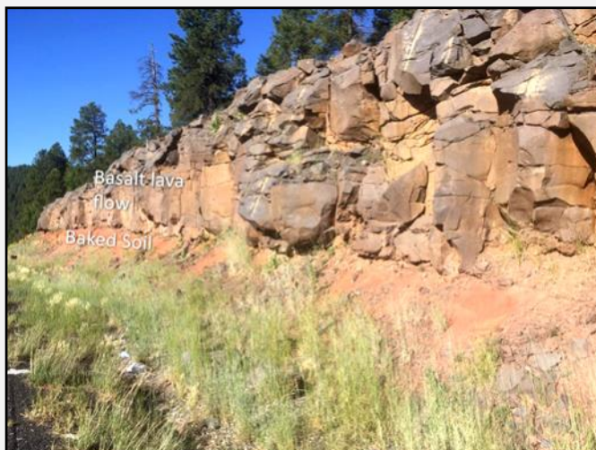
This is a view of a roadcut on I-17, about 10 miles south of Flagstaff. The baked soil and basalt lava flow are labelled in white (look closely). Photo by Mike Conway and courtesy of the Arizona Geological Survey.
